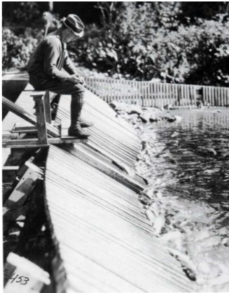
A weir across Anan Creek during the 1930s and 40s funneled returning salmon through a narrow opening. Above it sits a salmon counter from the U.S. Bureau of Fisheries. The counter is holding a "allywacker" or clicker to keep track of the number of fish passing up through the weir.
