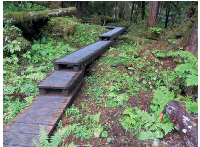
In flatter areas where the boardwalk steps gently like this example, gravel trail may be a suitable long term replacement.
