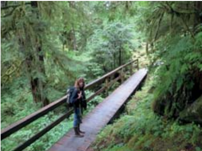
Typical raised boardwalk 3-feet wide with 2-rail railing on steep side.
