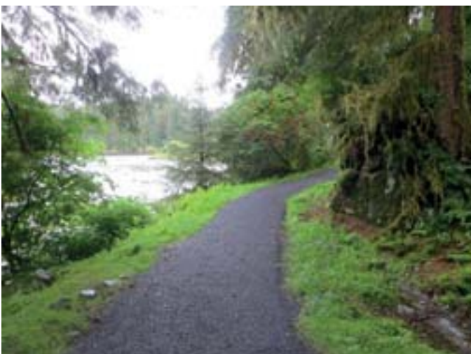
The 5-foot wide gravel trail was built on an area with an existing road base that was a relatively gentle grade. This location provides a good view of the creek near the lagoon.
