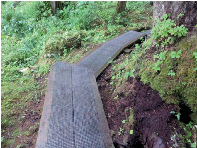
The trailhead to observatory trail has horizontal planking while the cabin to trailhead trail has longitudinal planking. Note wire mesh for non-slip surface.
