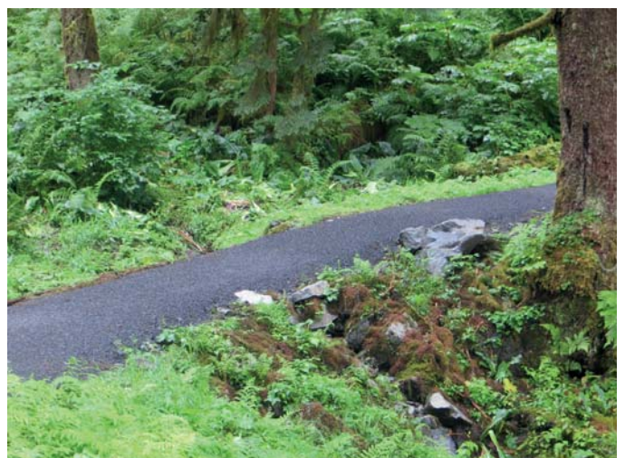
Drainage is conveyed beneath the trail in a culvert. the culvert is concealed with stone work and moss placement.
