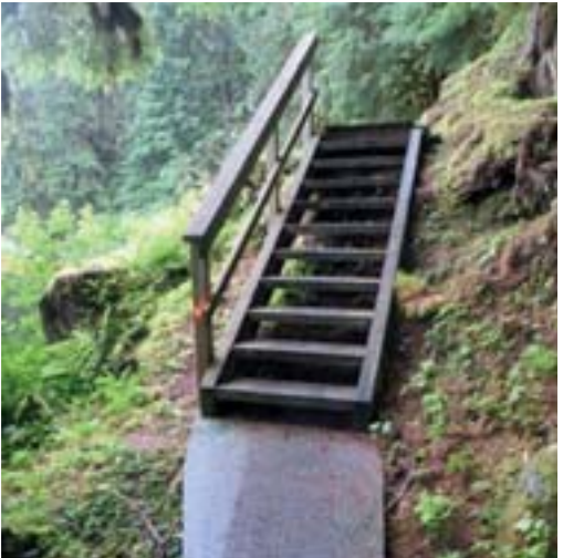
Typical staircase with treads supported on runners. Standard step height of 7 (or 8?) inches. Trail widens from 2 to 3 feet to meet stairs.
